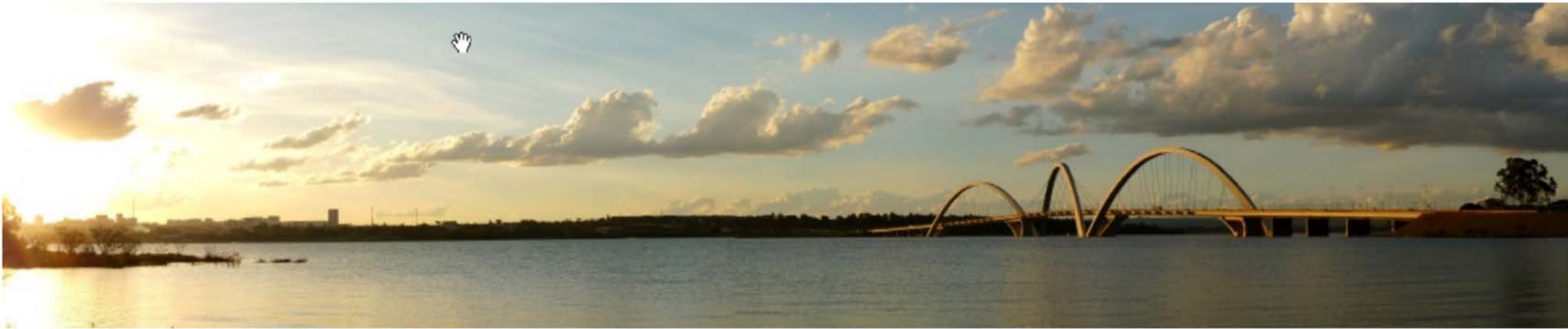
Juscelino Kubitschek Bridge Gigapan: Adonai Rocha
